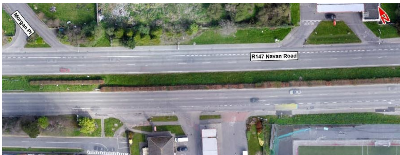
Image 6.16: R147 Navan Road / Morgan Place / Filling Station Junctions
