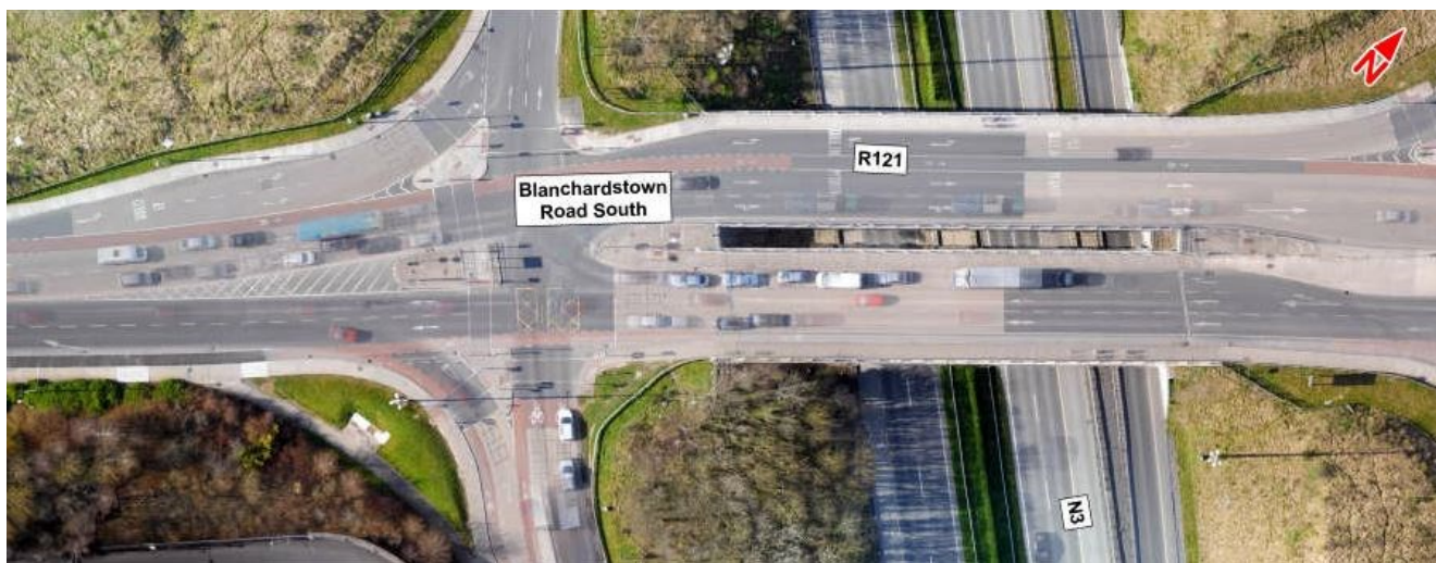
Image 6.3: R121 Blanchardstown Road South / N3 off-slip Signalised Junction
