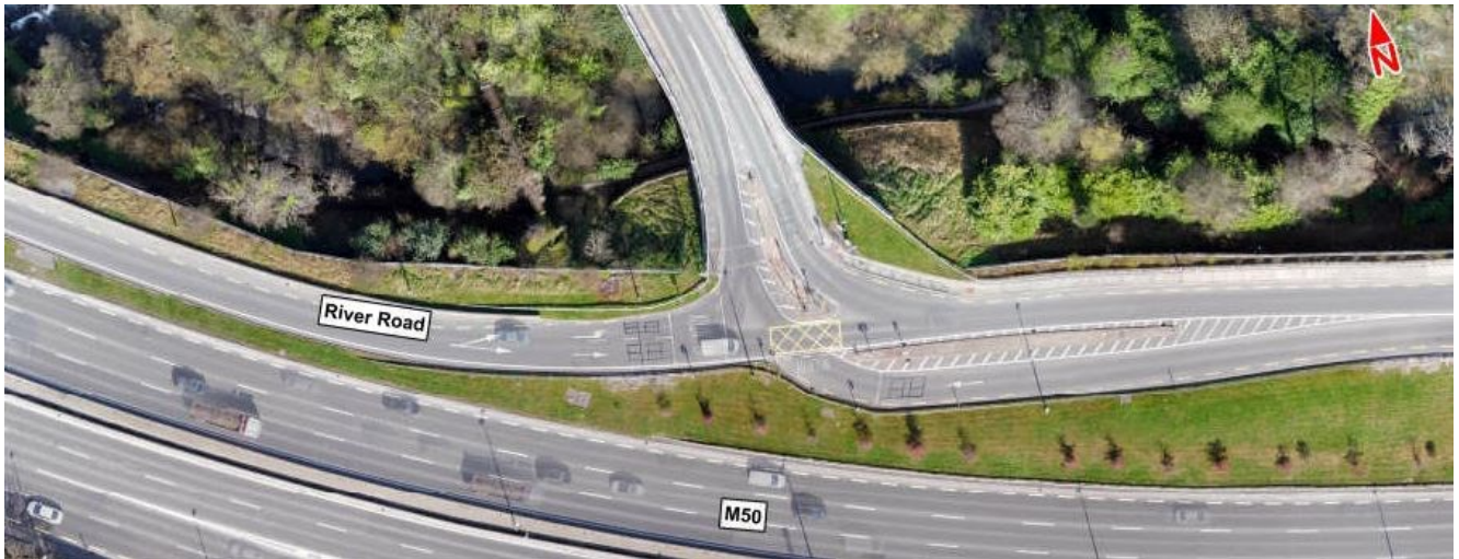
Image 6.11: N3 Eastbound off-slip (River Road) / Connolly Hospital Access Signalised Junction
