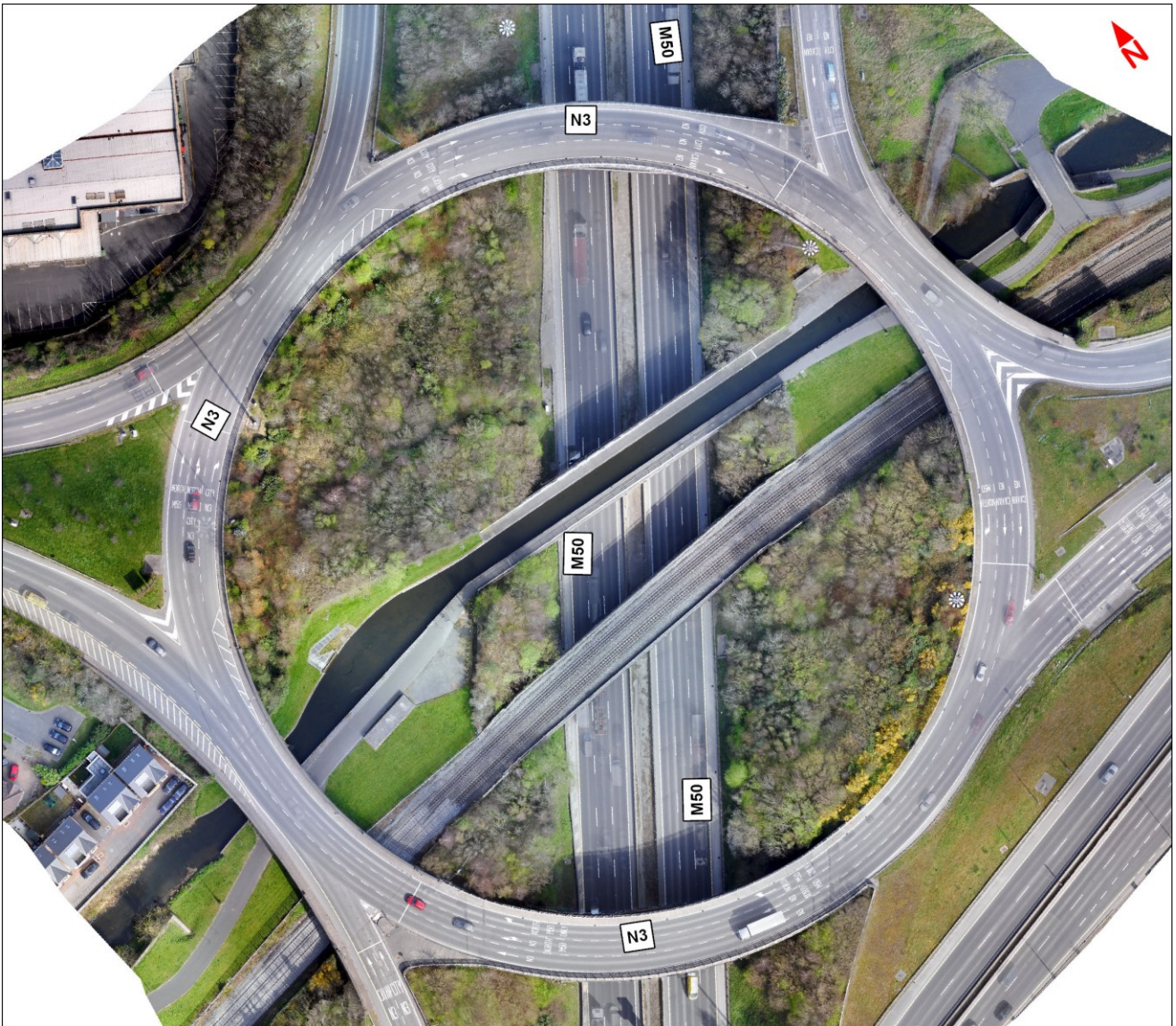
Image 6.14: N3 Navan Road / M50 Junction 6 Interchange
