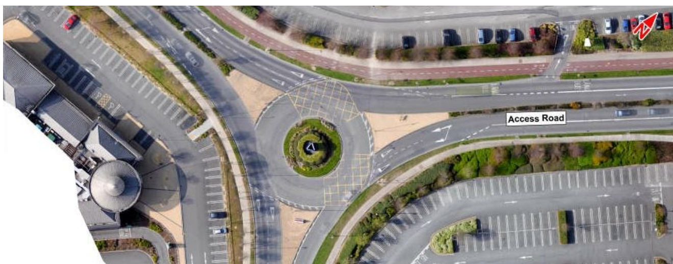
Image 6.7: Access Road / Access Road South Roundabout
