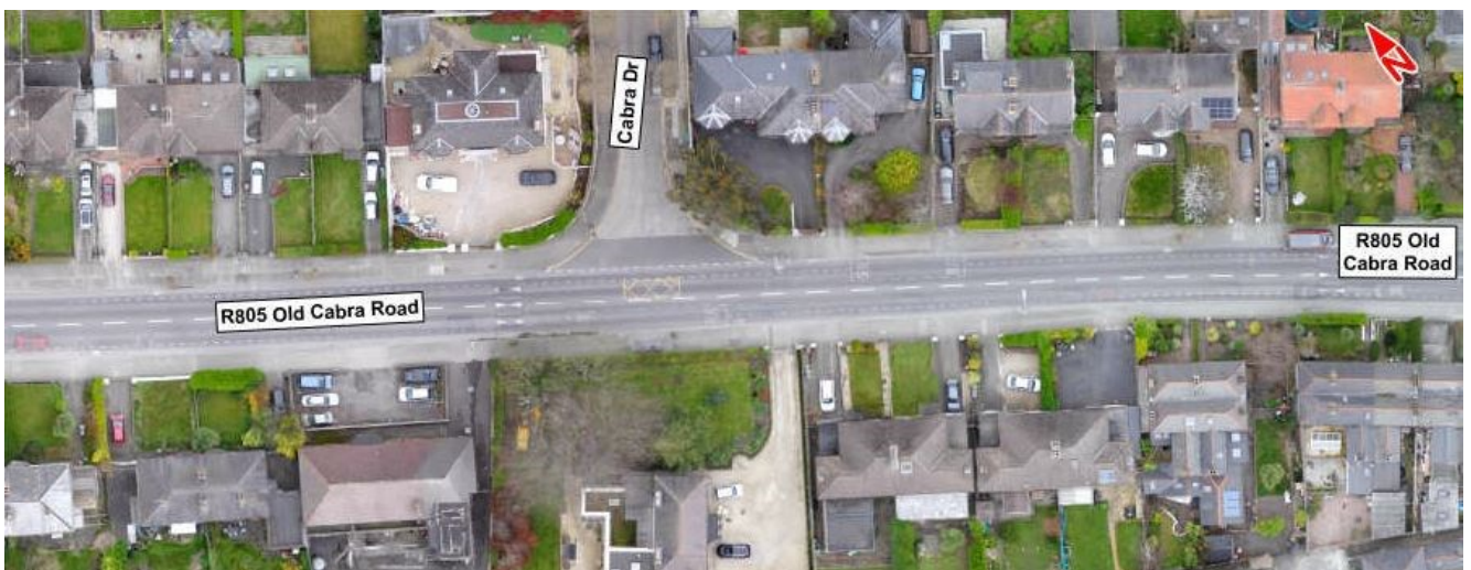
Image 6.29: R805 Old Cabra Road / Cabra Drive Priority Junction
