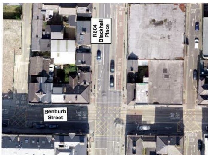
Image 6.39: Blackhall Place / Benburb Street Signalised Junction
